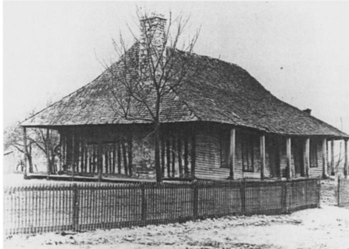
Fig 9 Poteaux-sur-solle Construction Cahokia Courthouse, a mid 18th century colonial building with close studded walls. Photo courtesy of Molly McKenzie, Illinois Historic Preservation Agency. (Source: from Jstor archive: <http://www.jstor.org/stable/20853104>.)
